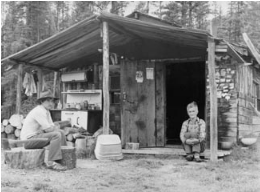
Trapper's cabin near Entrance AB
